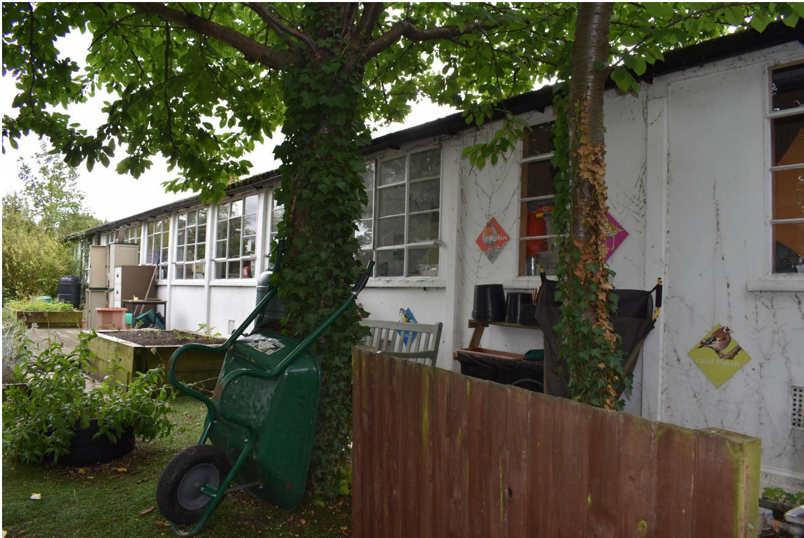
Plate 6: View across the rear of the building to be demolished (facing SE)
