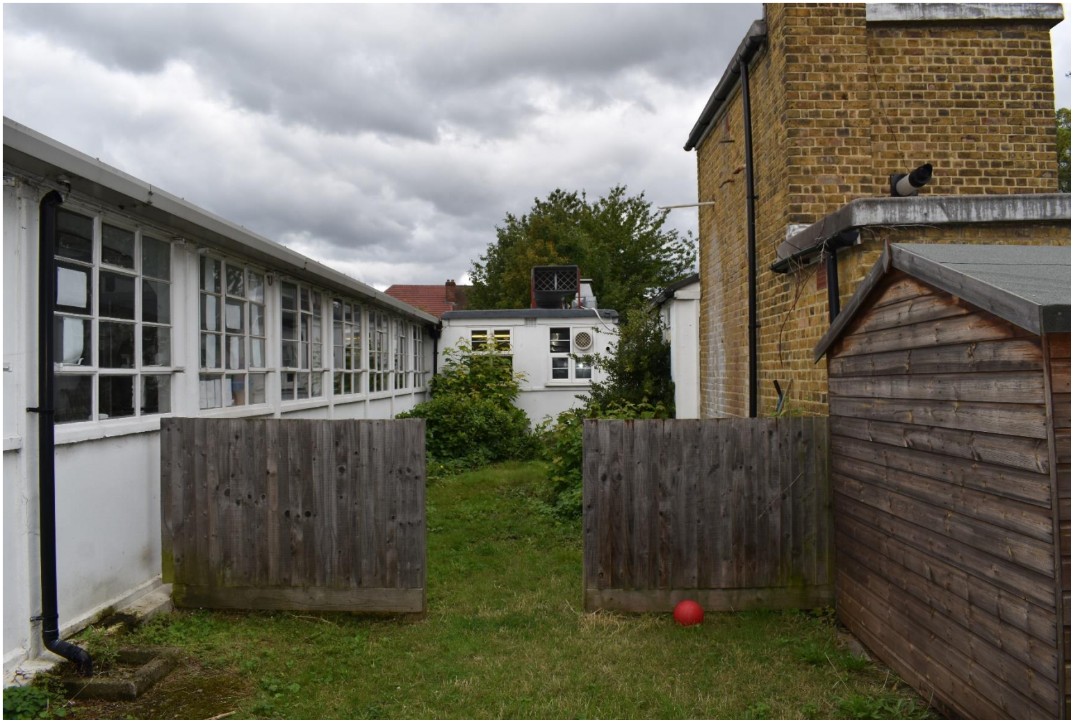
Plate 7: View of the area in between the building being demolished, west side (facing NW)
