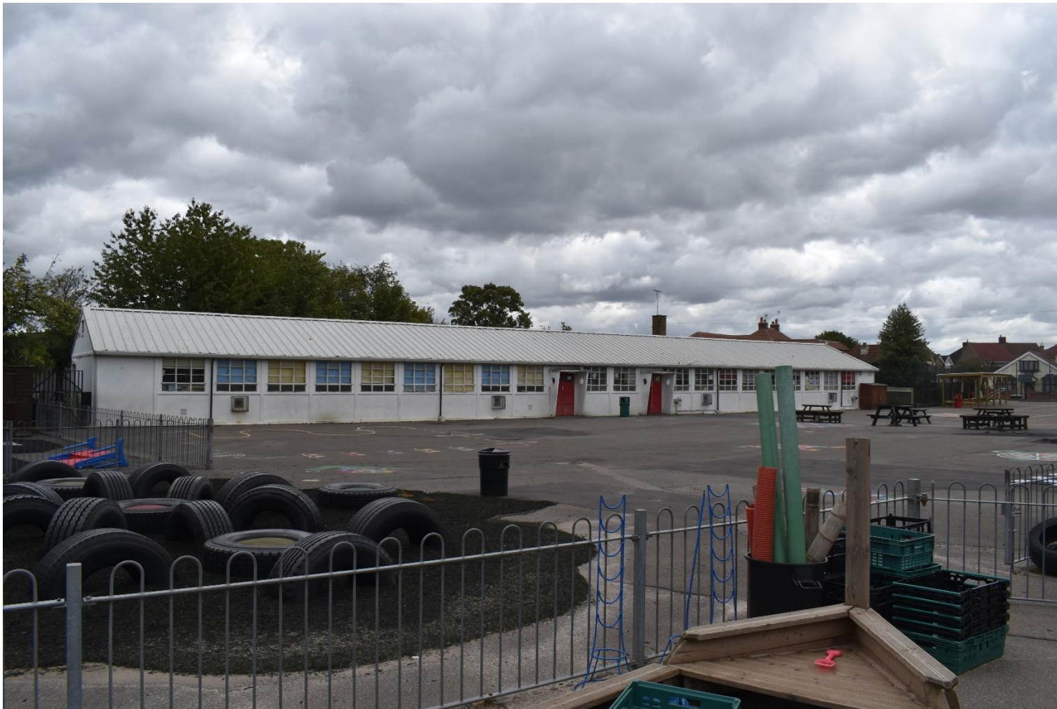
Plate 8: View of the front of the building being demolished from the playground (facing NE)
