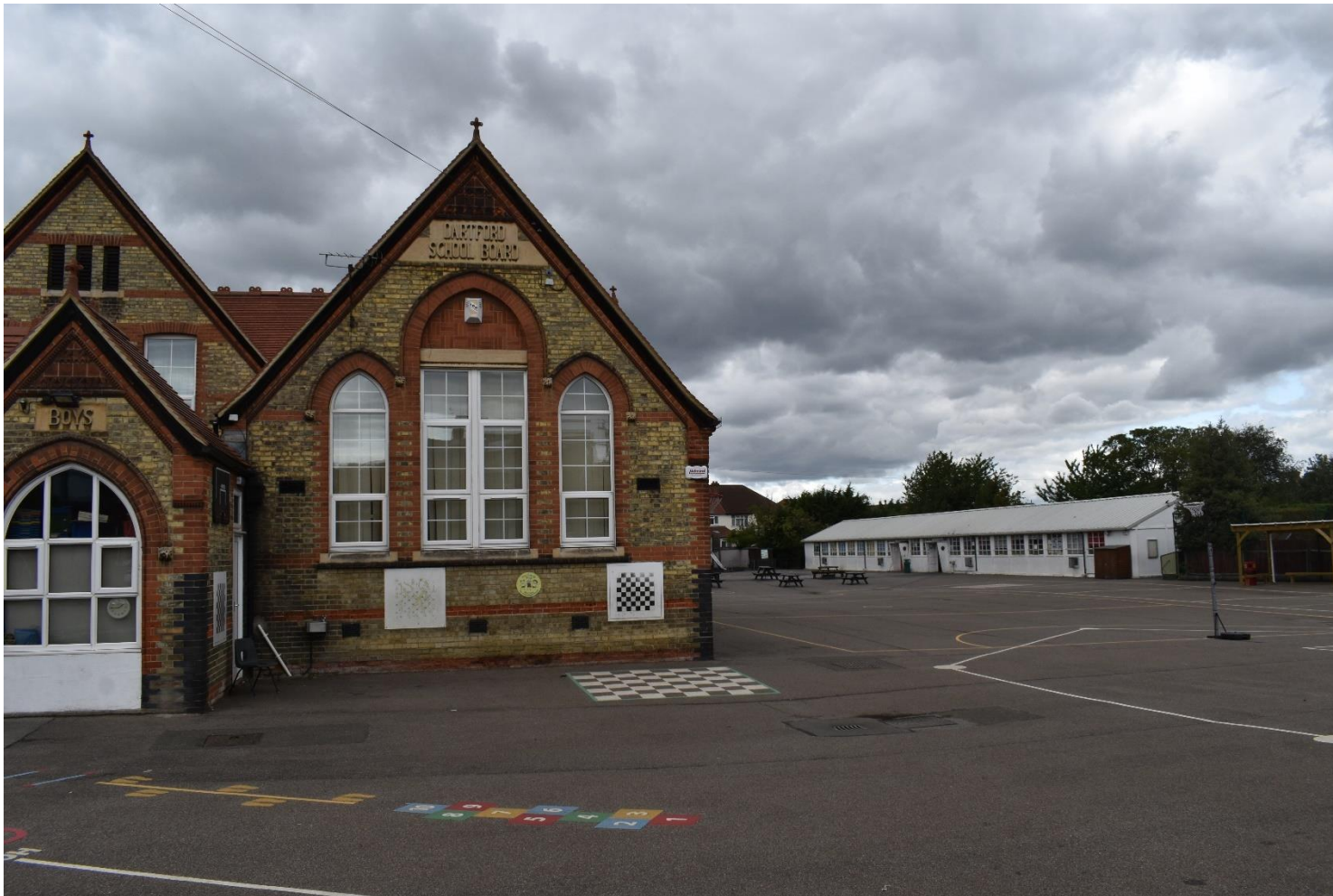
Plate 9: View the PDA across the playground (facing NW)
